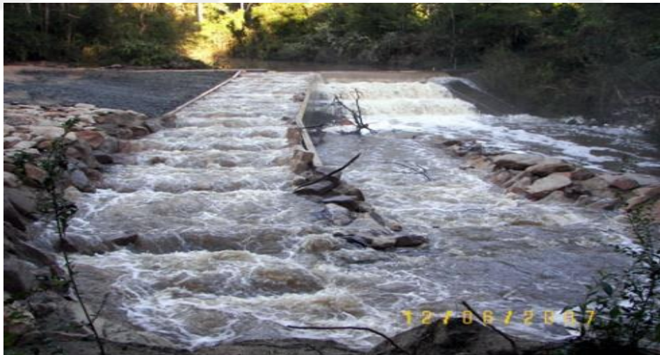
Figure 1.1 A Simple weir.
