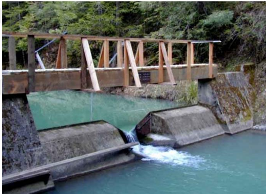
Figure 1.13 V-notch sharp crested weir.
