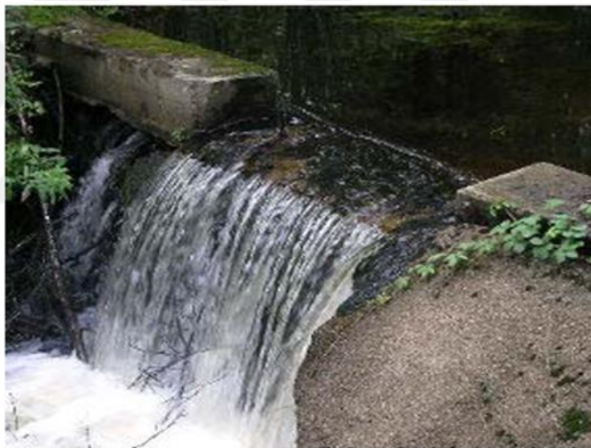
Figure 1.9 Broad crested weir in the field.
