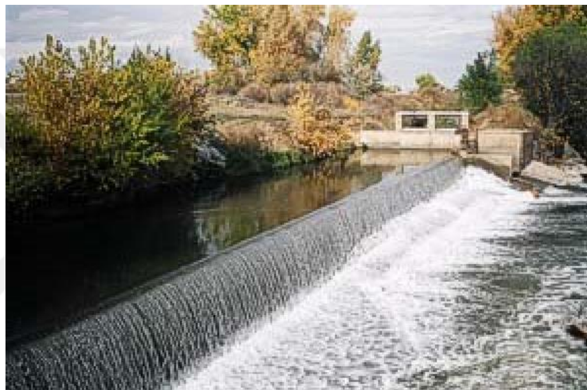
Figure 1.11 Sharp crested weir in the field.
