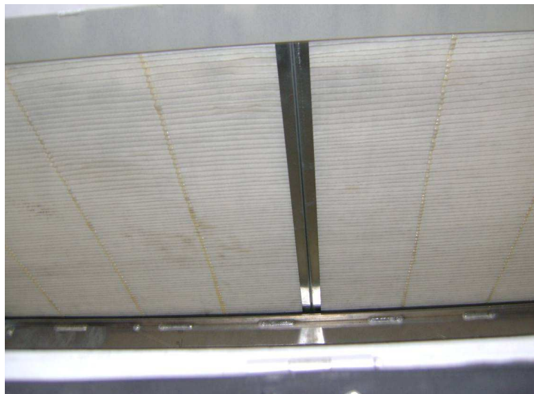
Figure 51 Inside of the Trash Container and Filters
