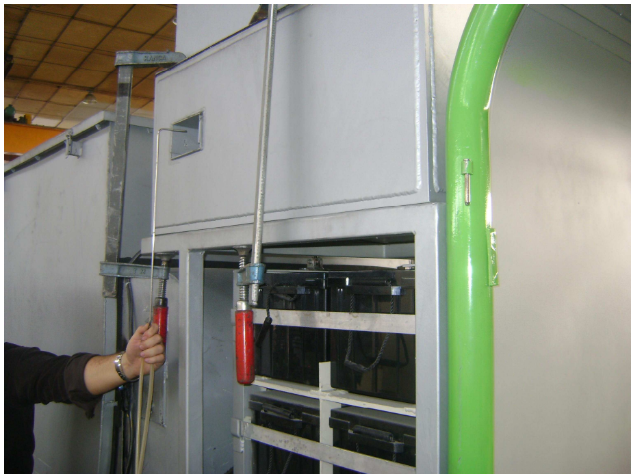
Figure 79 Measuring Air Speed at Fan Outlet with Pitot Tube
