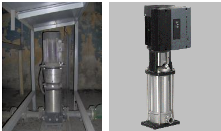
Figure 6.5 CRNE 32-4 A-F-G-E HQQE pump
