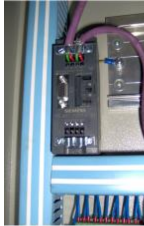
Figure 6.9. Repeater for regenerating the signals in amplitude and time.
