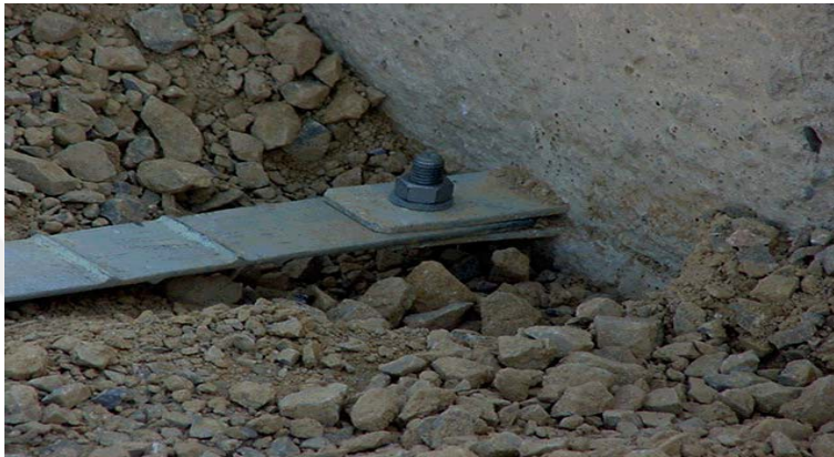
Figure 5.1 : Connection parts in steel strips (Ekli, 2006).
