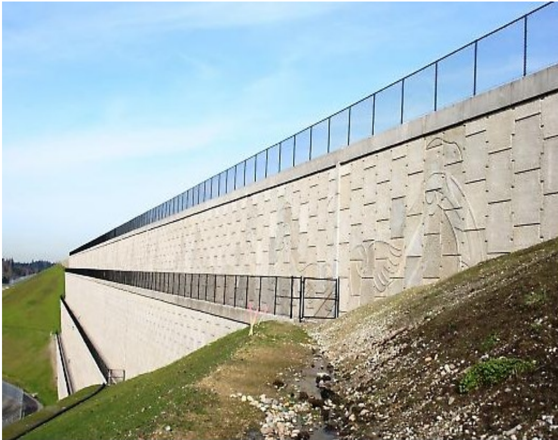
Figure 5.3 : Sea-Tac Airport - 3rd Runway, WA-reinforced earth company (Reinforced earth company, 2009).
