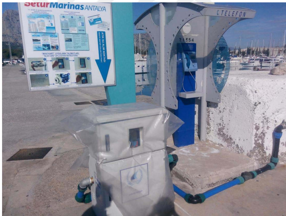
Image 2. Blue Card System for Bilge Water Discharging
