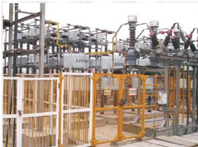
Figure 4.20 Filter Banks of SVC
