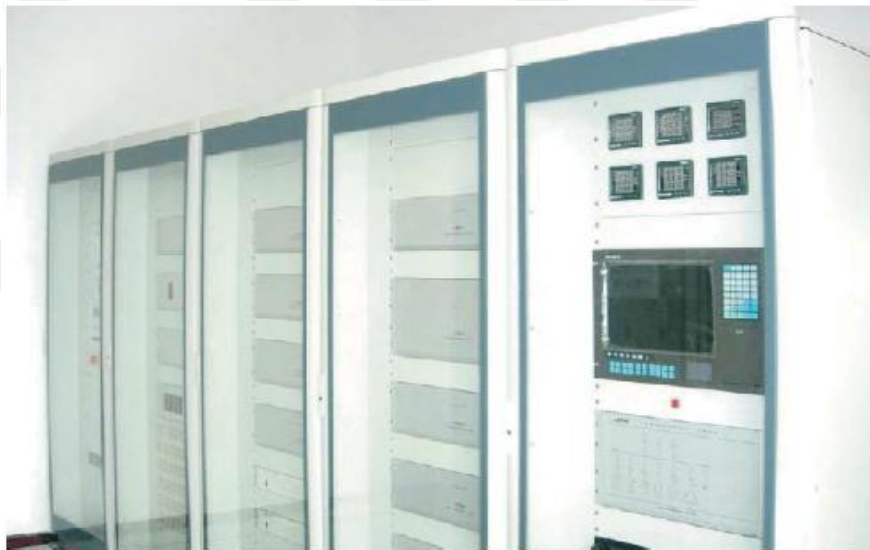
Figure 4.16 Control and Protection System of SVC
