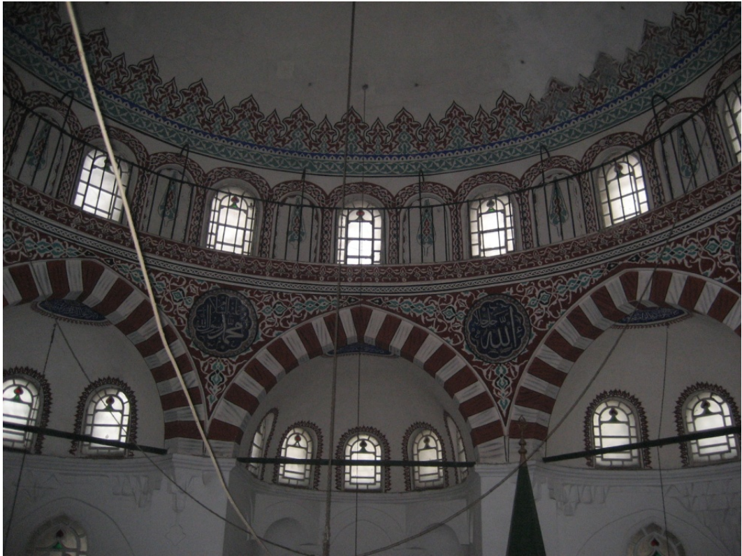
Figure 5.7: Mosque interior; arches, tromps, pendentives and arch ties
