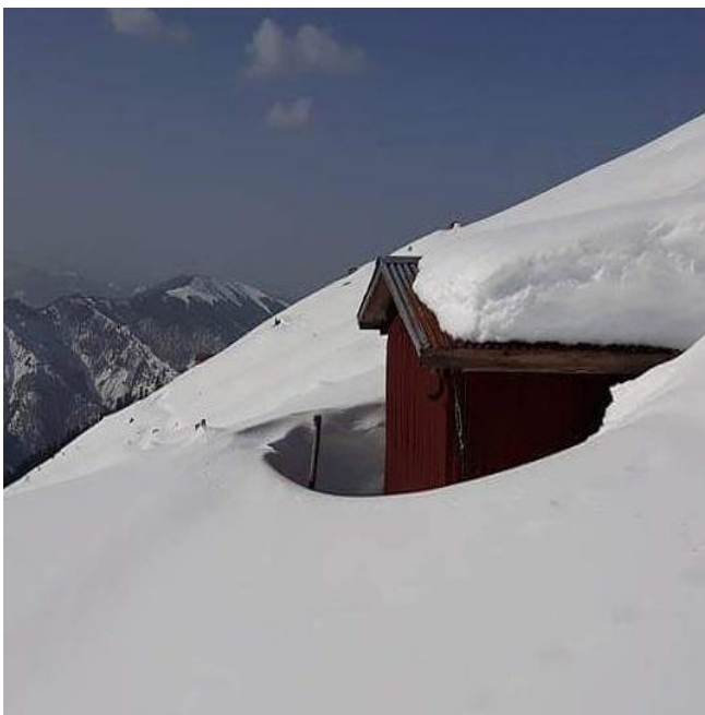
Figure 17: A house at avalanche starting area
