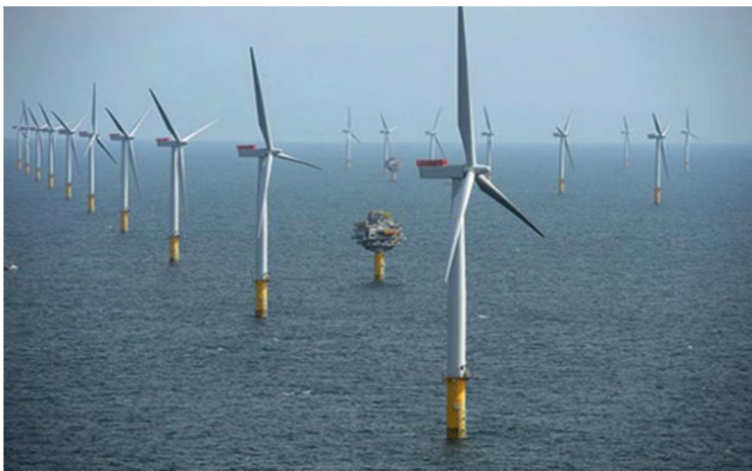
Figure 2.2: Wind power plant.
