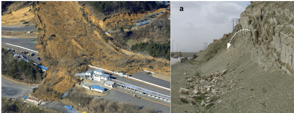
Figure 2.1 Example of a landslide and a toppling failure
