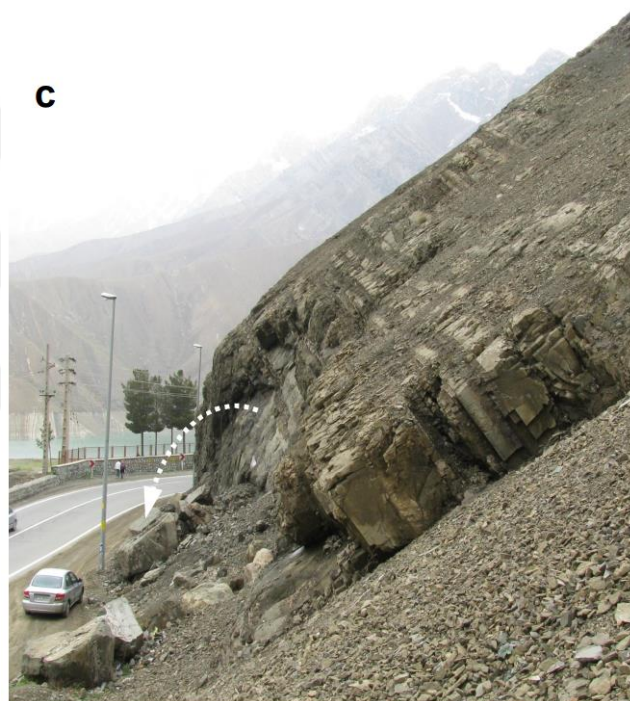
Figure 1.2 Toppling failure close to the road
