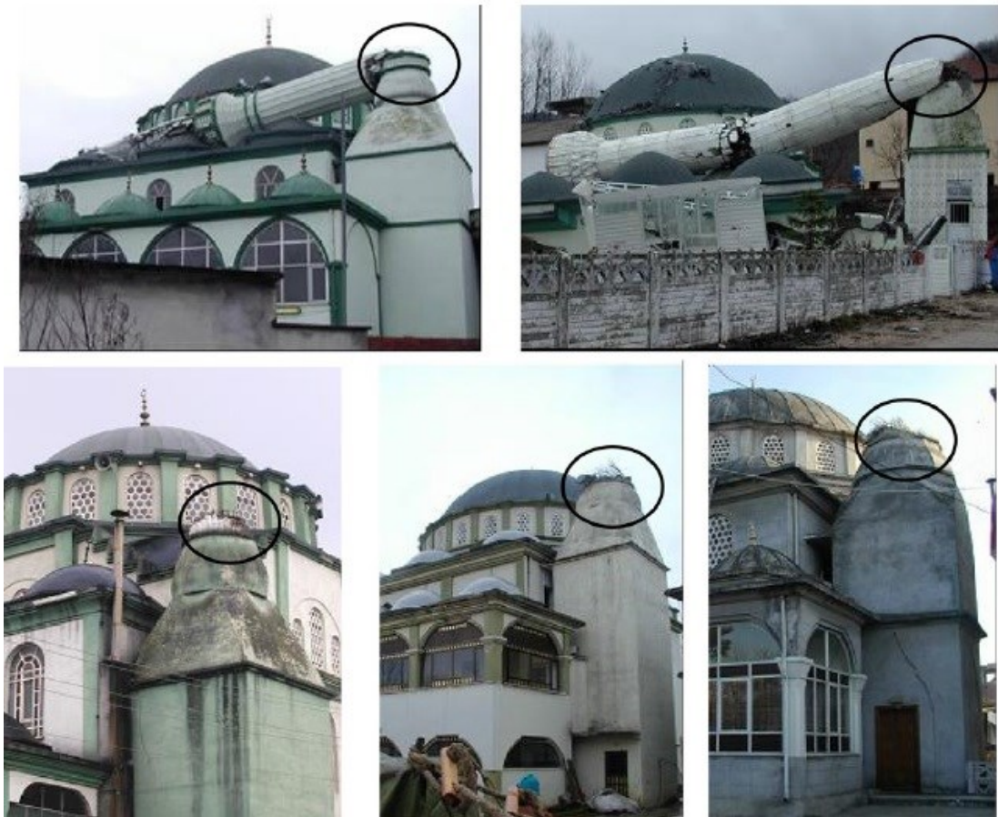
Figure 1.7: Minaret failures near the bottom of the cylinder bodies.
