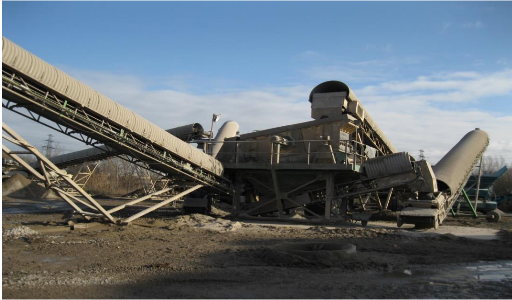
Figure 3.25 : Overlooking of the recycling plant at Arkenberge in Berlin.
