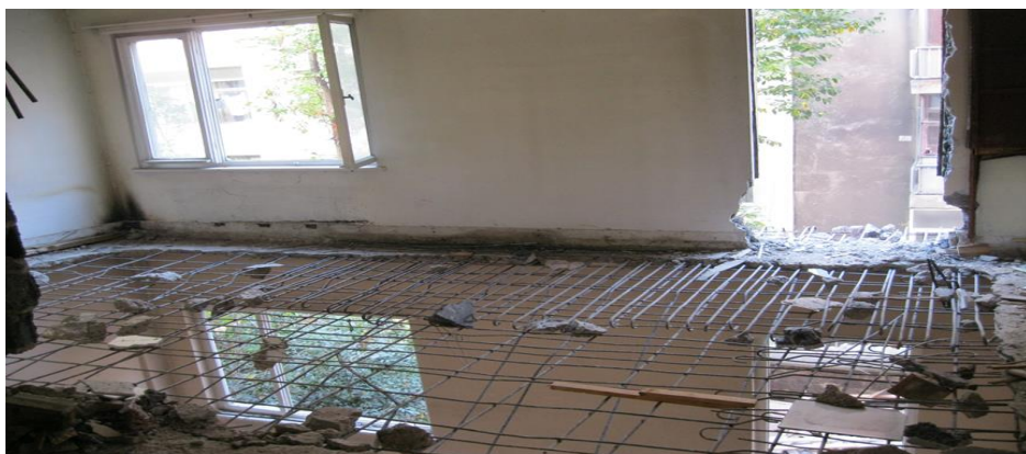
Figure 3.11 : Dismantlement of balconies.
