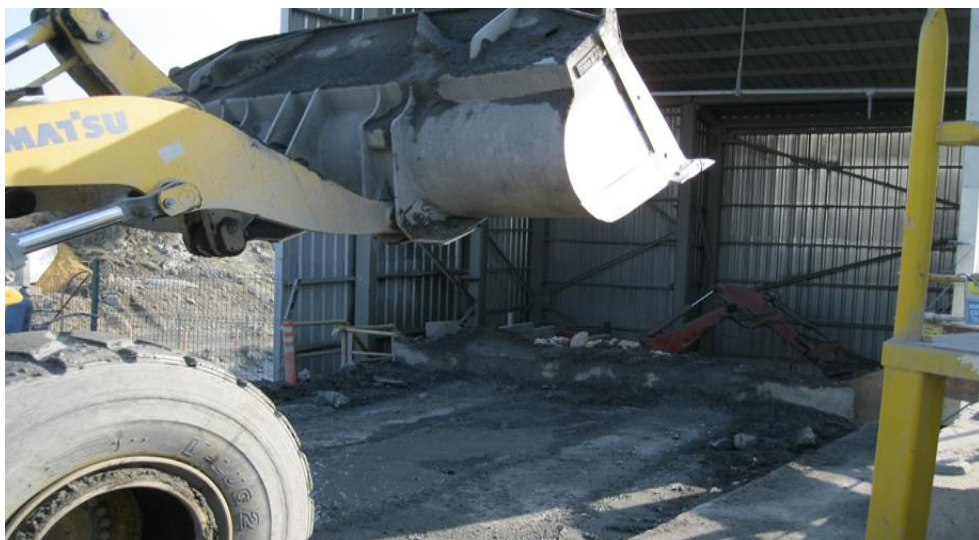
Figure 3.20 : Transportation of demolition waste to the hopper of the jaw crusher.
