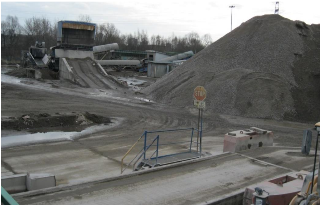
Figure 3.26 : The hopper of the crusher at Arkenberge in Berlin.
