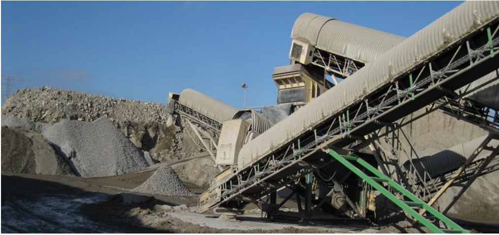
Figure 3.29 : C&D waste and RCA at the recycling plant at Arkenberge in Berlin.
