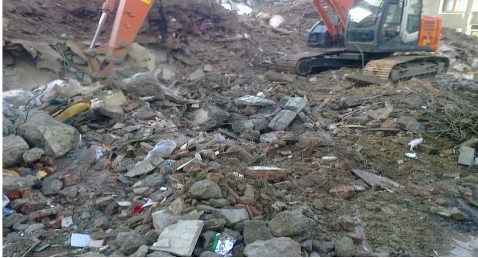
Figure 3.14 : Last step of mechanical demolition.
