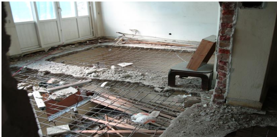
Figure 3.10 : Dismantlement of interior walls.
