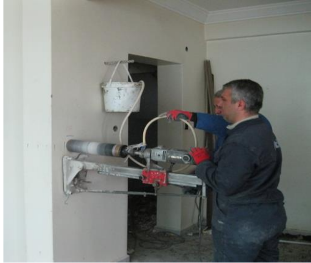
Figure 4.5 : Taking core sample from the building.
