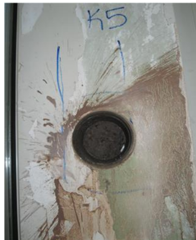
Figure 4.6 : Taking out the core from the column.
