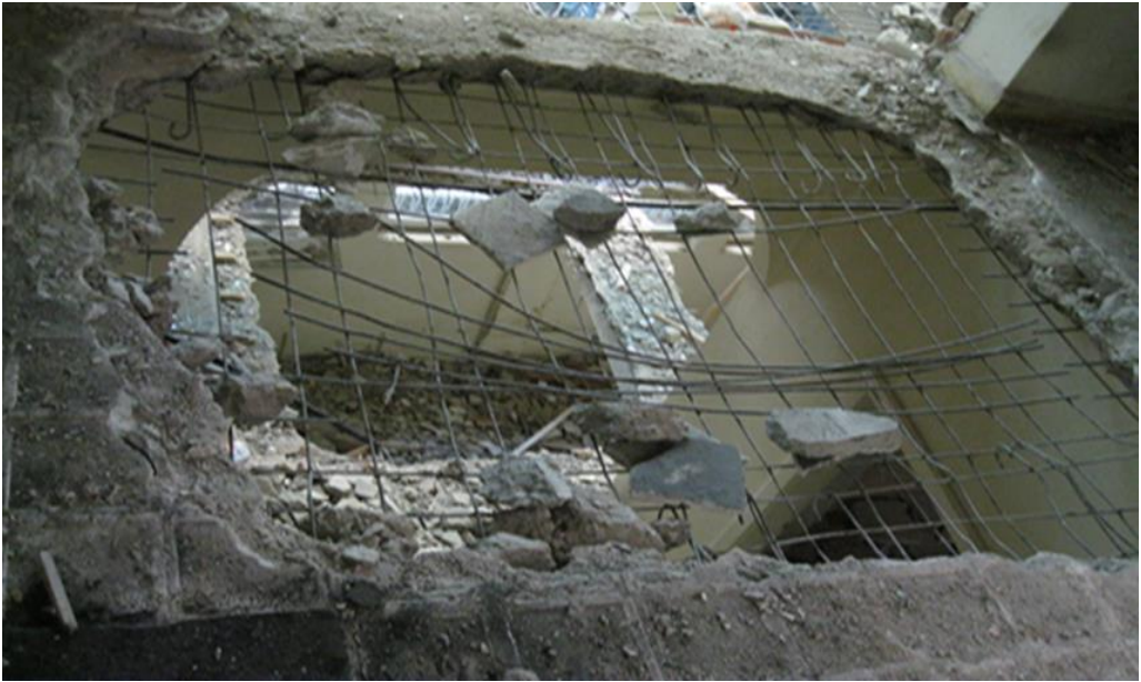
Figure 3.8 : Hand demolition on every floor of the apartment.
