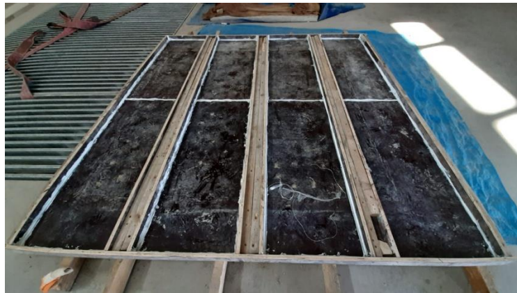
Figure 21: Formworks
