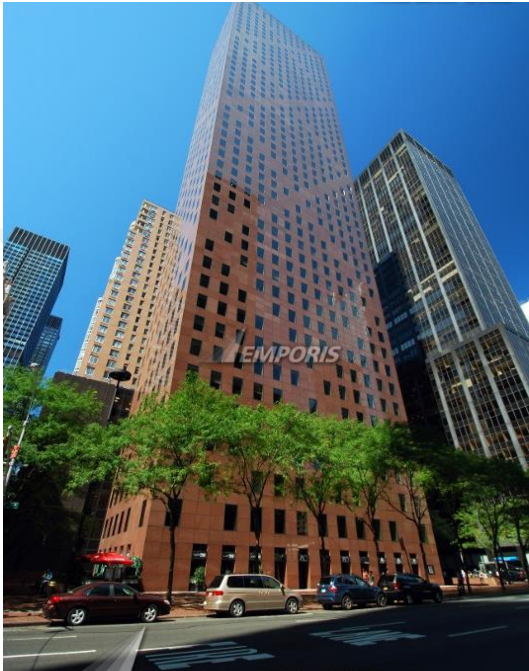
Figure 2.28 The 780 Third Avenue Building, New York, USA, 1985 (Gunel and Ilgin, 2006)
