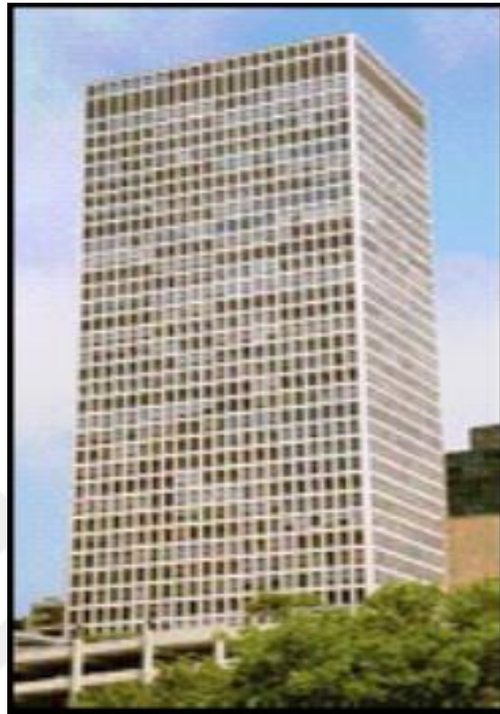
Figure 2.23 Framed Tube (Gunel and Ilgin, 2006)
