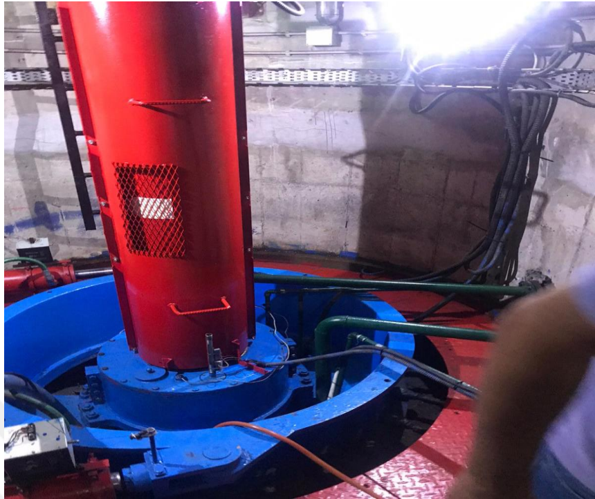
Figure 3.1. Kaplan turbine.
