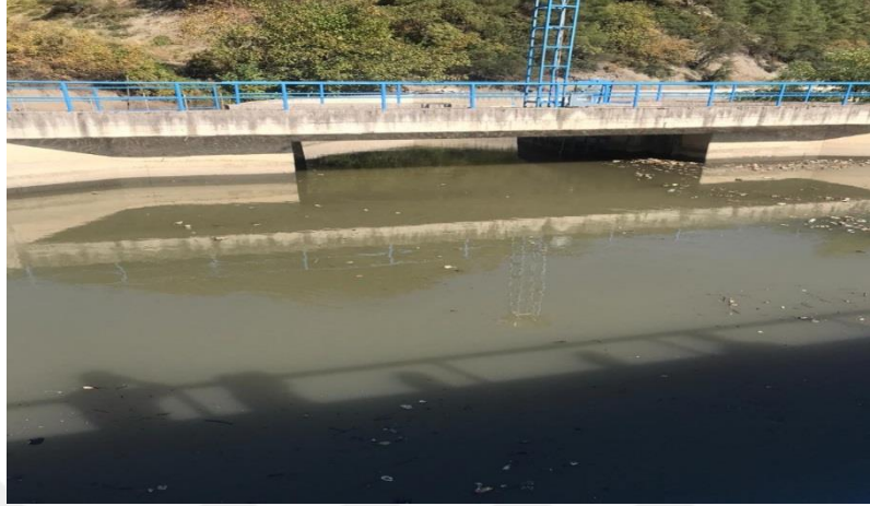
Figure 4.3. Forebay of RRHPP.
