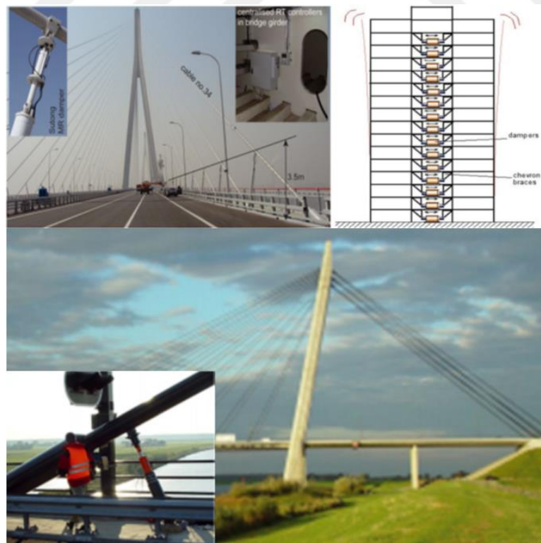
Figure 1.23: MR dampers in infrastructures for vibration absorber during earthquakes [90,95]
