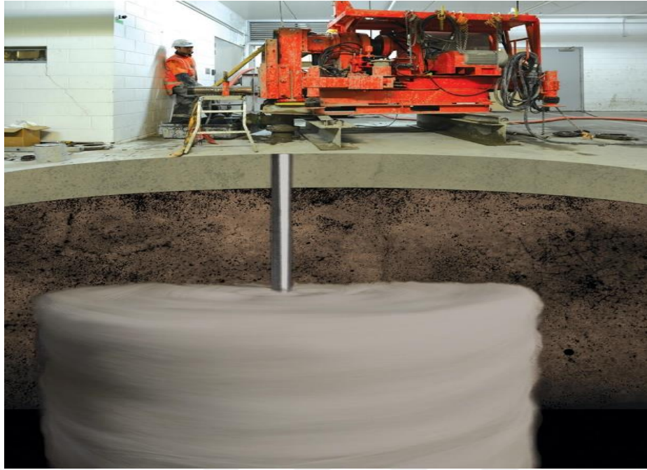
Figure 2.11 Jet injection method
