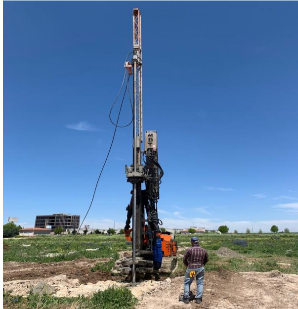
Figure 3.15 Jet grouting of dry river sand soil
