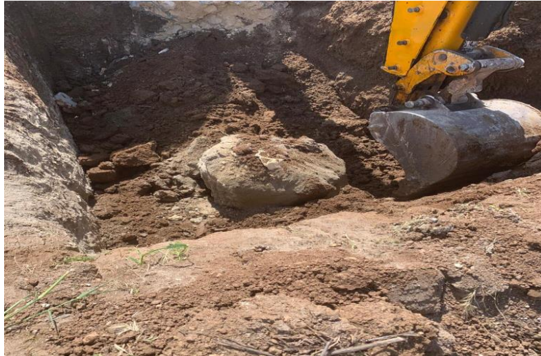
Figure 3.17 Excavation around of Jet grout column
