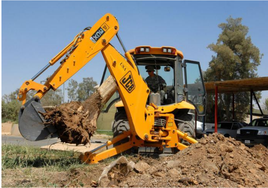
Figure 3.3 Picture of Excavation Machine
