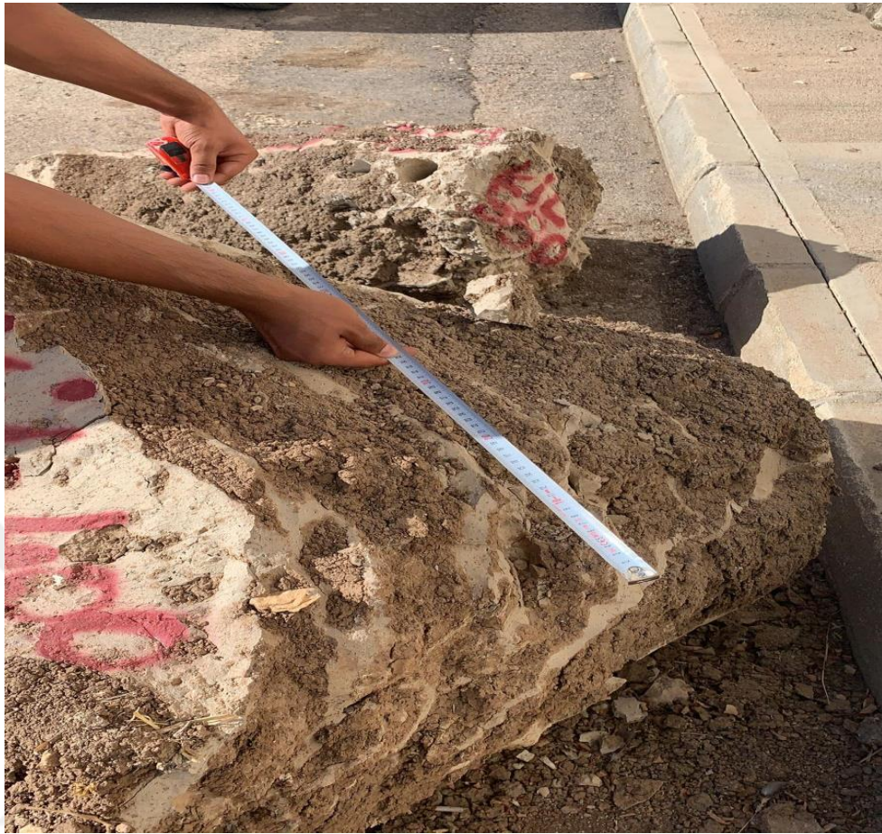
Figure 4.1 Measure of jet grout columns diameter
