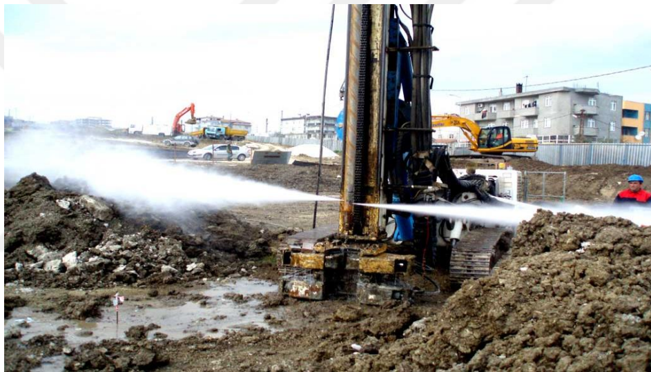
Figure 2.12 Jet grout
