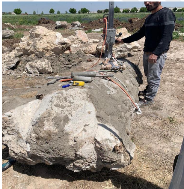
Figure 3.18 Taking coring samples on jet grout
