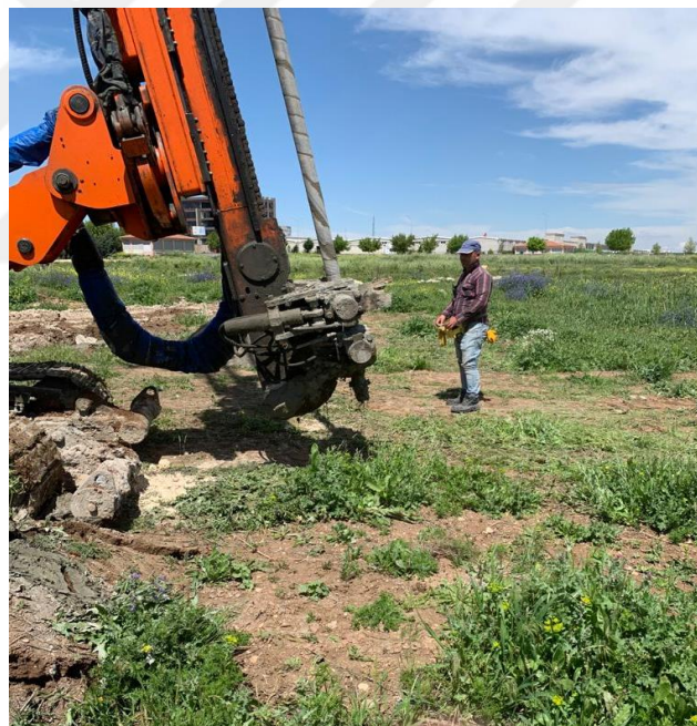
Figure 3.16 Jet grouting of clay soil
