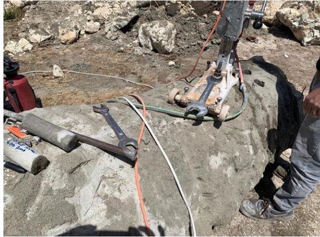
Figure 3.19 Taking coring samples from Jet grout columns
