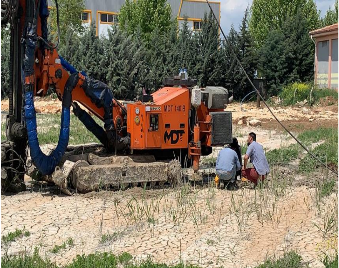
Figure 3.11 Jet grout testing machine
