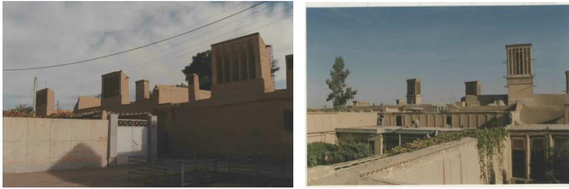
Figure 5.10. (continue ) Left, an ordinary wind catcher Ardakan, Iran, right, a (four sided wind catcher in Yazd, Iran) Two types of wind catchers in the old quarter of the cities of central Iran. above, one directional towers in Ardakan, blow four directional towers in Yazd (Mahyari, 1996).
