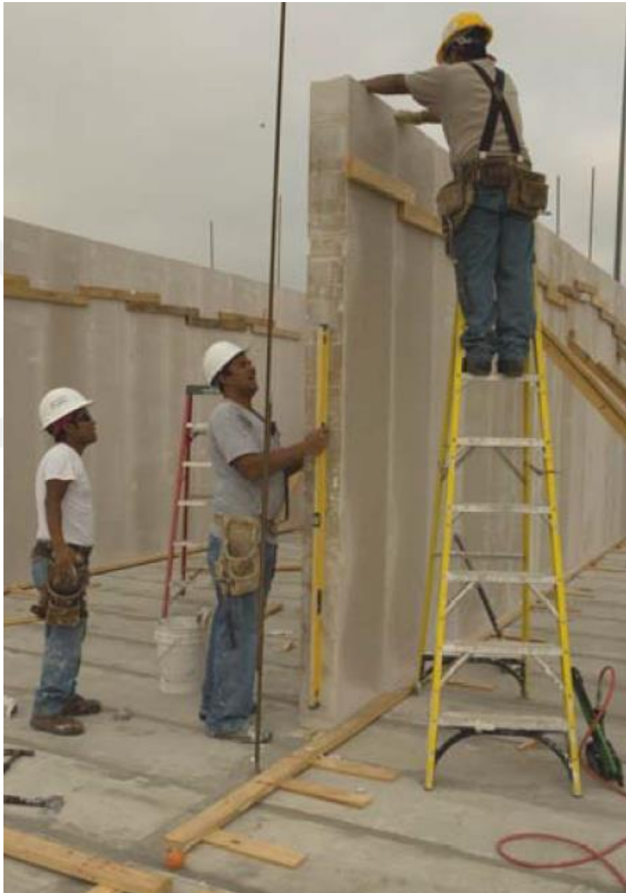
Figure 1.12: Placement of Panel with a Level (Xella, 2010)
