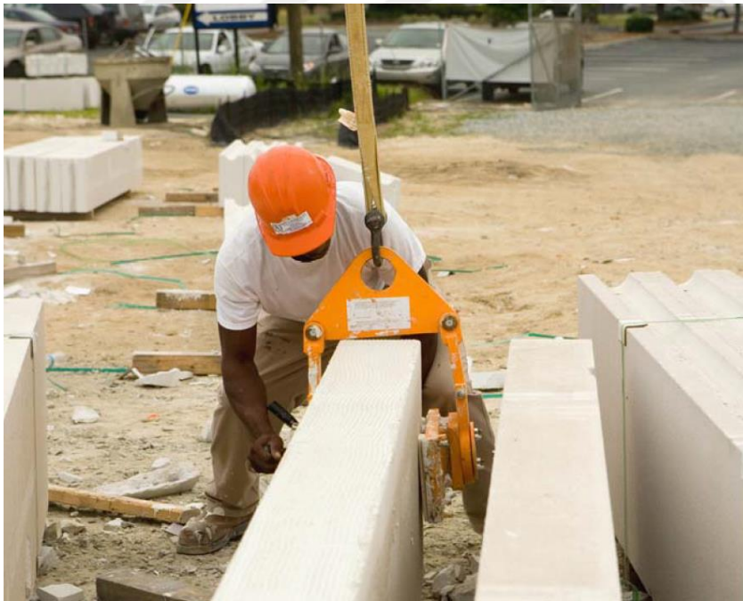
Figure 1.11: Lifting of AAC Panel (Xella, 2010)
