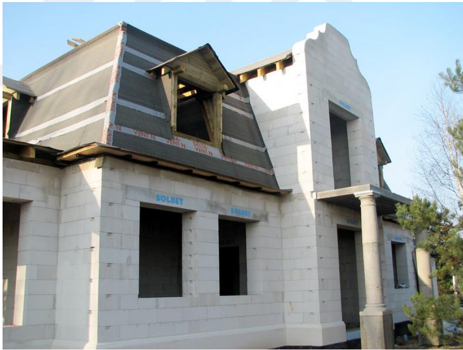
Figure 1.10: Use of AAC blocks and lintels (Myanmar Business, 2017)
