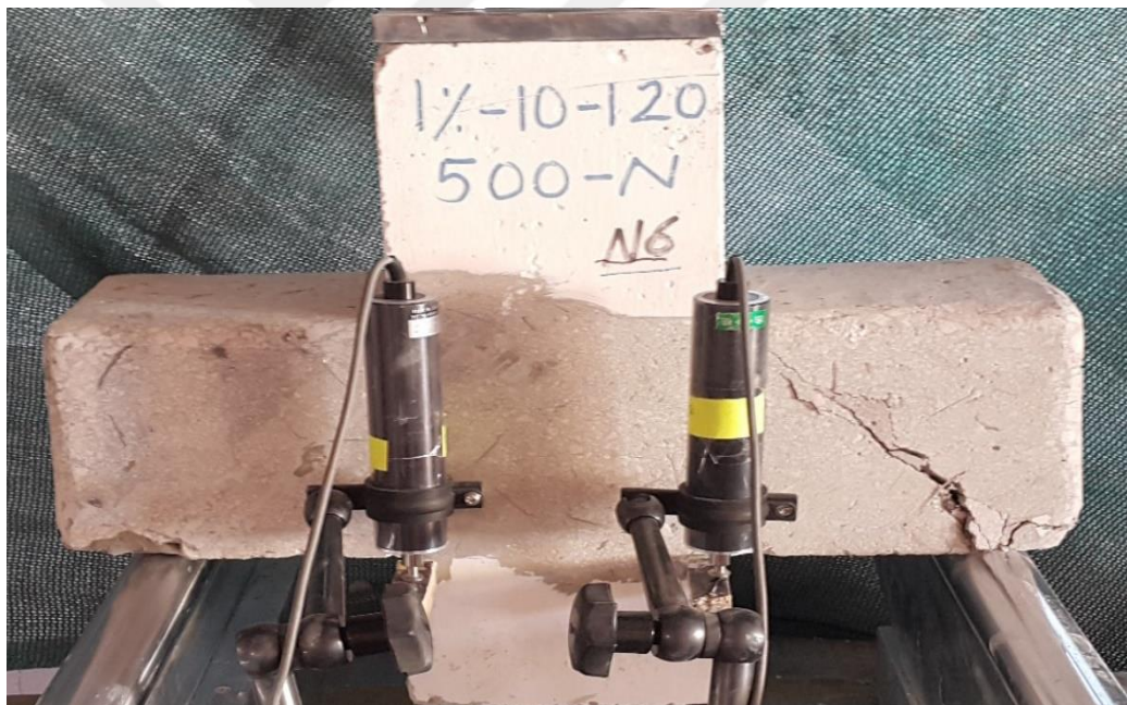
Figure 4.24 Specimen (C8-1.0-500 ) failure after repairing
