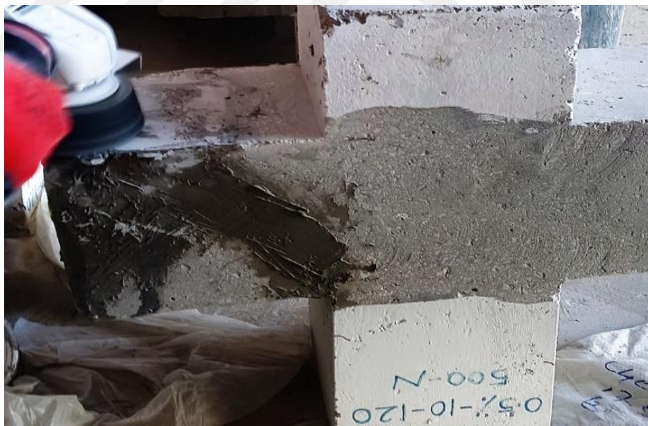
Figure 3.10 Grinding after injection
