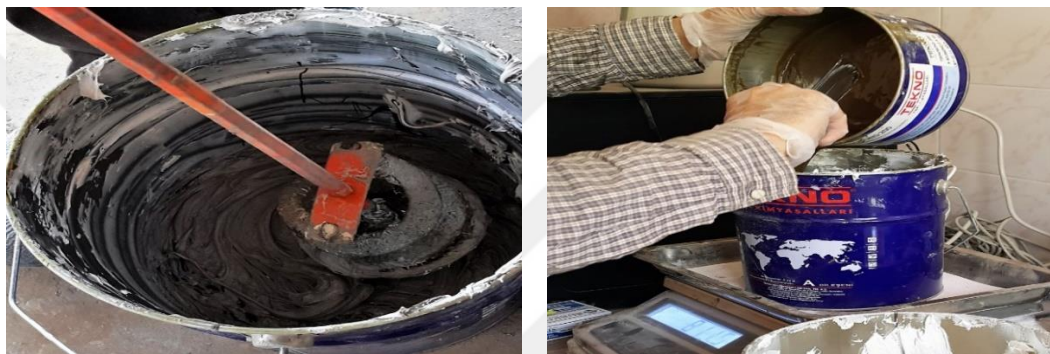
Figure 3.7 Mixing of high viscosity epoxy
