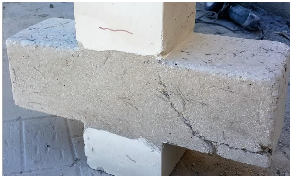
Figure 3.4 Low damaged corbel
