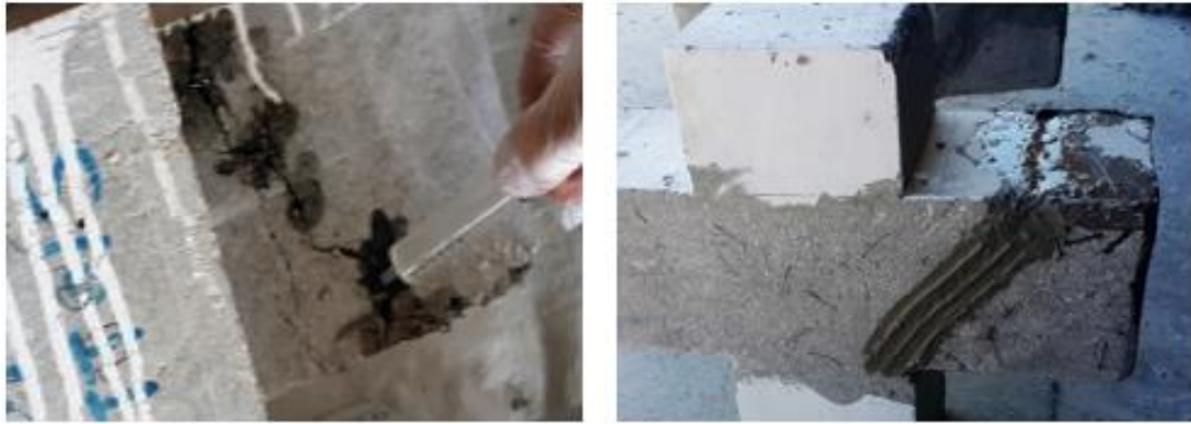
Figure 3.9 Crack repair epoxy(Sikadur-52) injection
