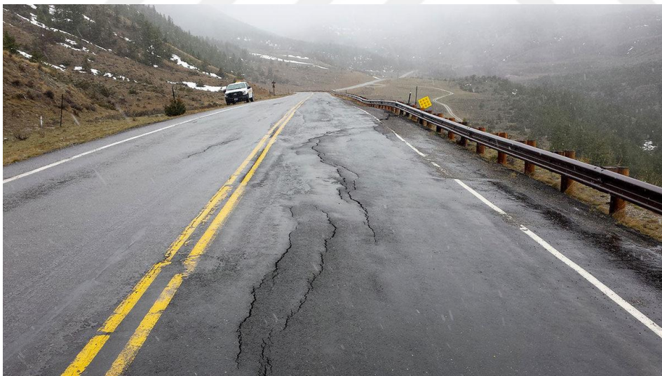
Figure 2.2. Cracks on a highway surface which are caused by rainfall induced minor landslides on the highway embankment (Adopted from www.codyenterprise.com )
