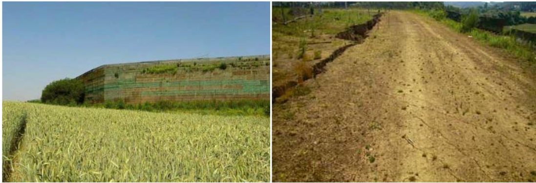
Figure 2.3. A tensile crack behind reinforcement zone of a retaining wall which is made from reinforced soil (Vanicek, 2013)
