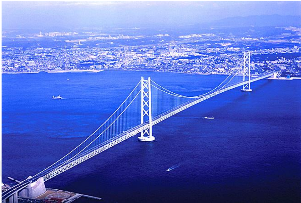
Figure.2.1 Akashi-Kaikyo Bridge in Japan (Google, 1998)
