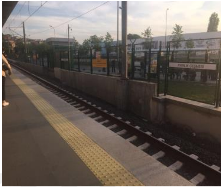
Picture 10. Ayrilikcesme Metro Station [Source: Author, April 2016]
