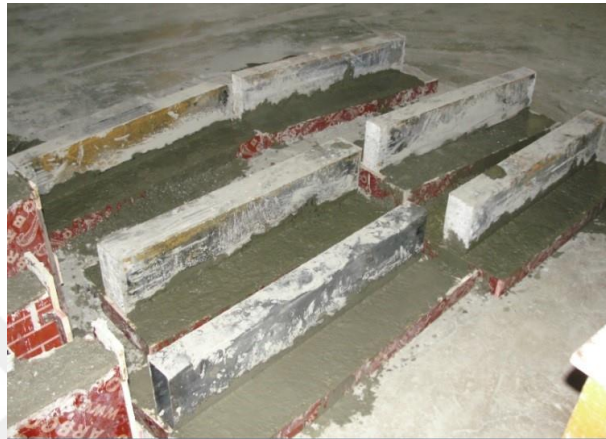
Figure 3.8 Casting of the concrete deck slab
