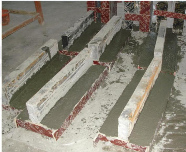
Figure 3.14 Casting the plywood formwork for the concrete slab
