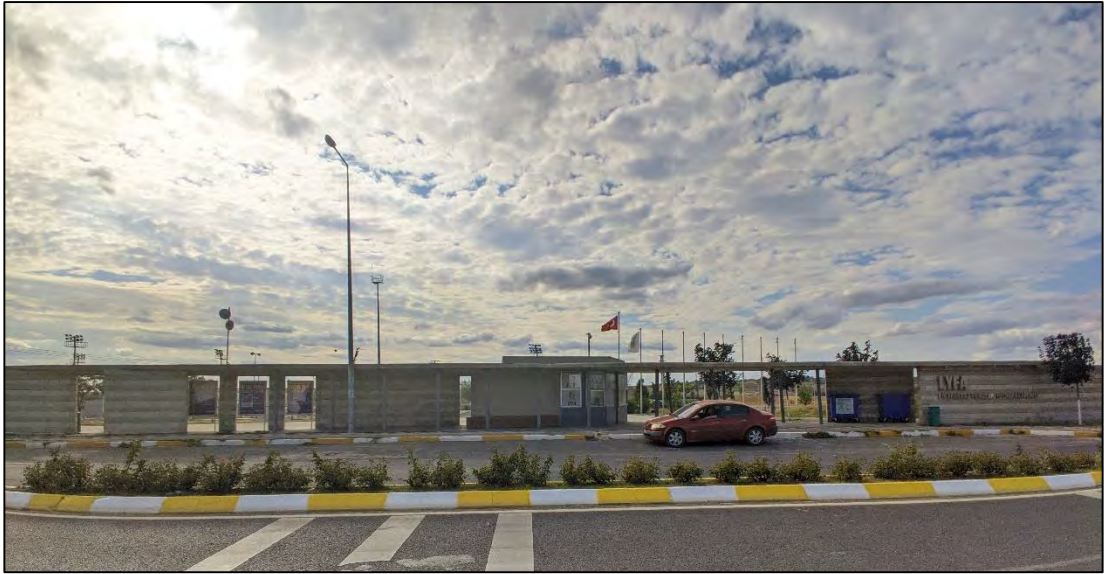
Figure 16: Entrance view of LYFA
