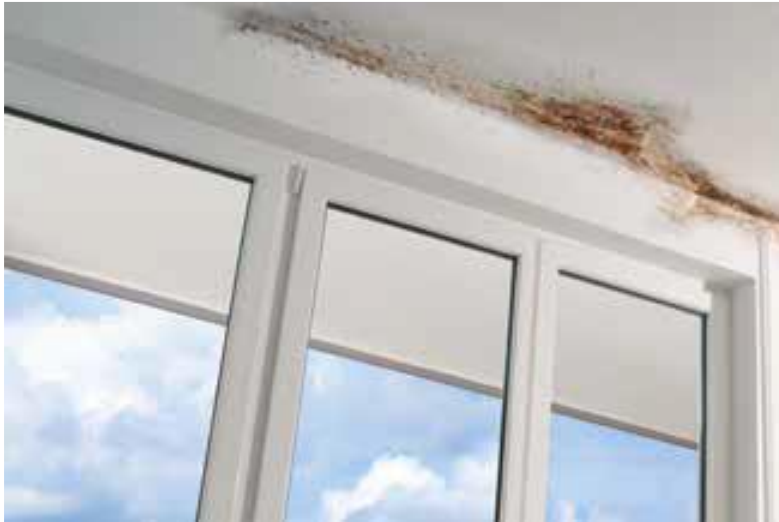
Figure 2.2. Photograph showing mould growth on the ceiling of a concrete slab adjacent to an exposed slab edge thermal bridge. Condensation forms here frequently as a result of colder interior surface temperatures. ( https://www.schoeck.com/en-gb/structural-thermal-bridges ).
