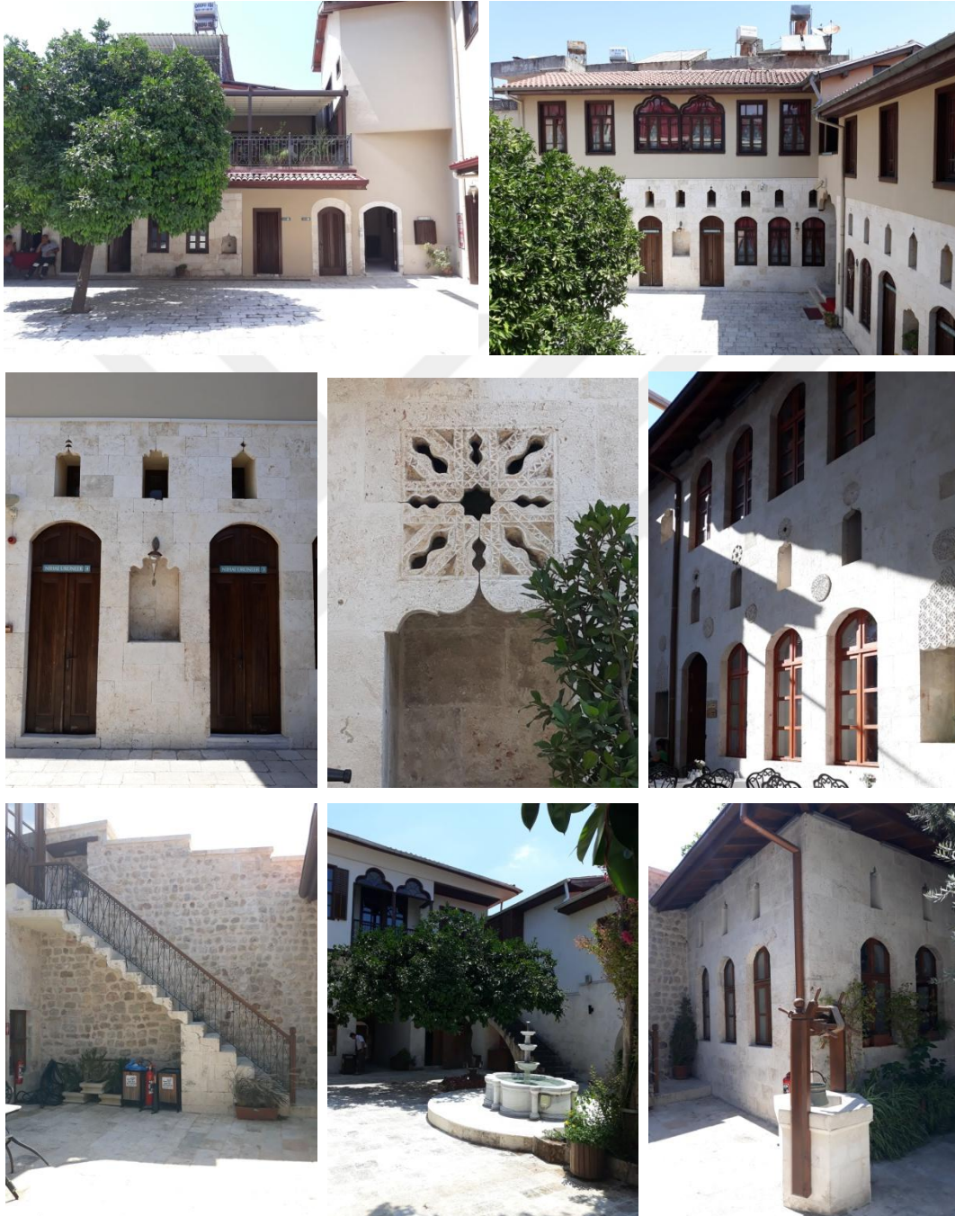
Figure 4.42. Some sections of the house and the courtyard (taken from the author's personal archive)
