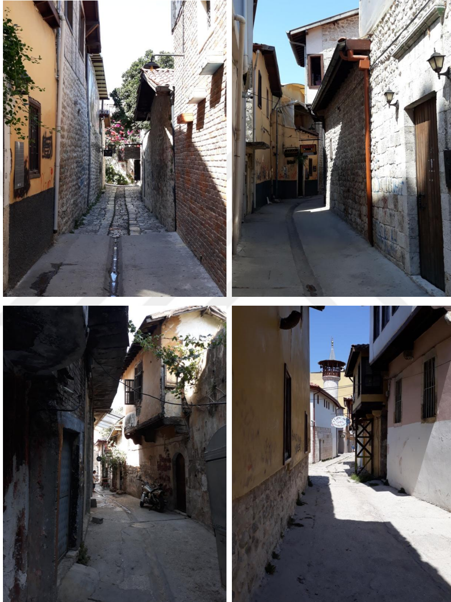
Figure 4.37. Some sections from the streets of old Antakya (taken from the author's personal archive)
