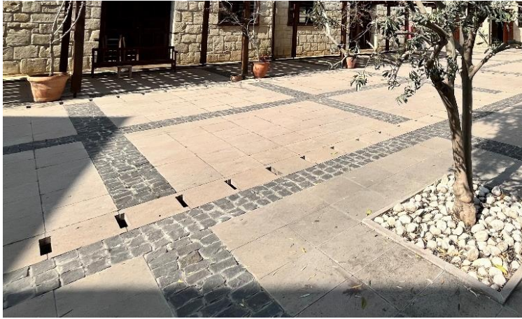
Figure 53. New perforated Floor for rainwater drain of the courtyard
