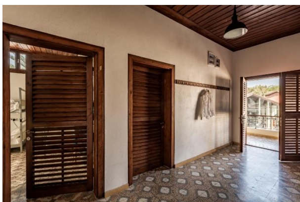
Figure 48. Louvered Doors of the Building D, First floor view (Source: SAYKA, 2025)
