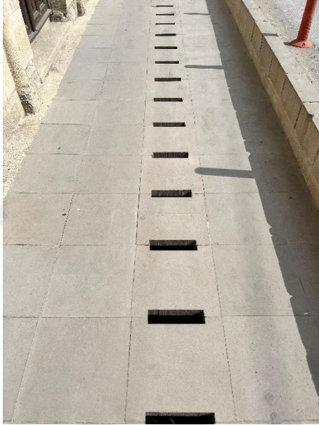
Figure 51. Hollow Slabs for the collecting rainwater
