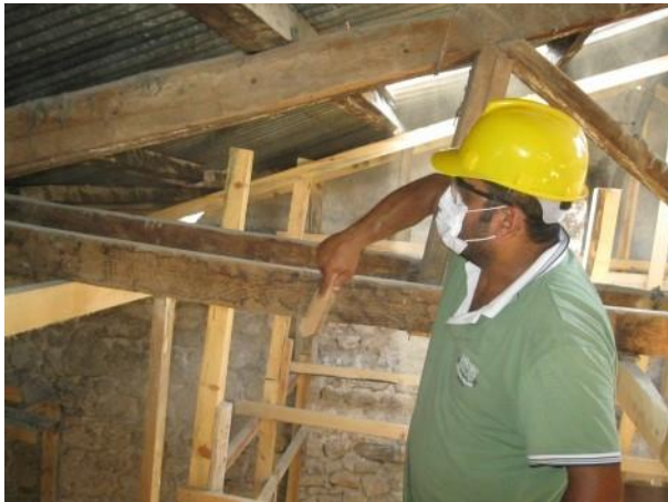
Figure A. 4. Cleaning process of the wooden trusses with bristle brushes (Source: SAYKA, 2025)
