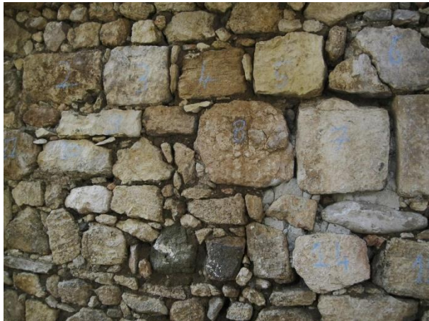
Figure 38. Numbered Stones (Source: SAYKA,2025)
