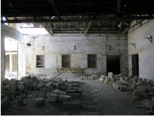
Figure 37. Interior Stone walls with the finishing of Cement-Based Plaster (Source: SAYKA,2025)
