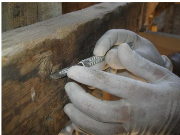
Figure A. 6. Restoring Wooden Trusses (Source: Arkiv,2025)
