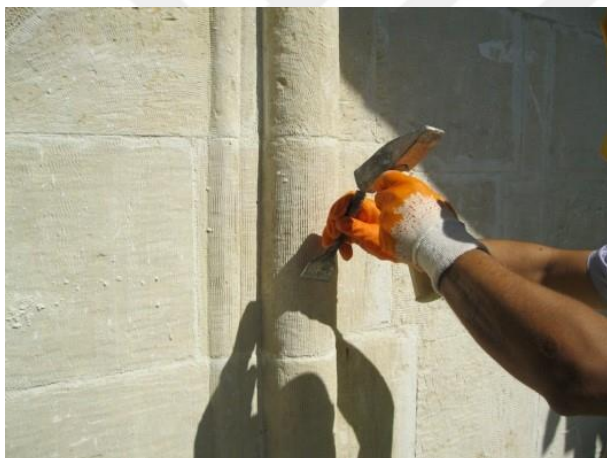
Figure A. 3. Giving different texture to the new stones with hammer (Source:SAYKA,2025)
