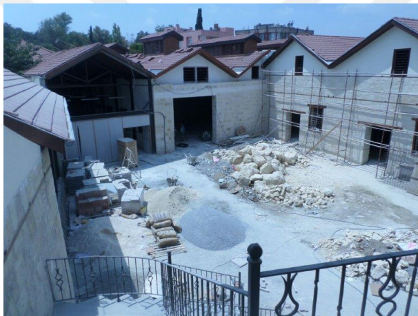
Figure 39. Restoration of the stone walls (BOUN,2025)
