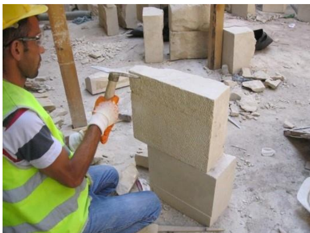
Figure A. 2. The process of crushing the stones brought to the building area in whole form in accordance with their original dimensions (Source: SAYKA, 2025)
