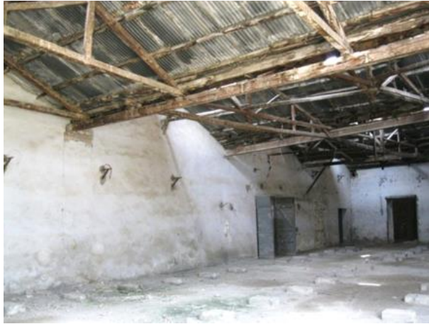
Figure 33. Cement-added plaster on the old walls of the building (SAYKA,2025)
