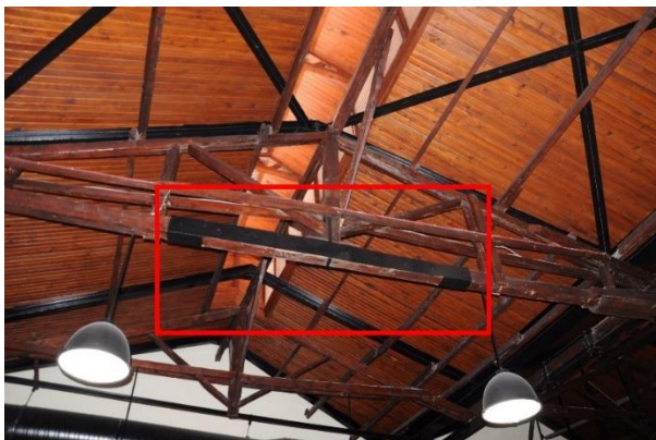
Figure 44. Addition of Steel elements for strengthening to the existing wooden trusses which originally carries the roof in the past
