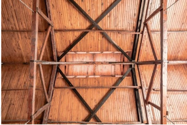
Figure 45. Newly added wooden ceiling coverings of the buildings (Source: SAYKA, 2025)
