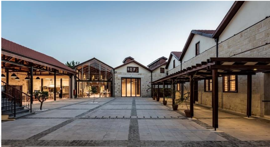
Figure 20. General overview of the complex from courtyard (Building A located at the end of the Picture, Building B and C located on the right side of the Picture and Building E located in the left side of the Picture ) (Source: Arkitera, 2025)
