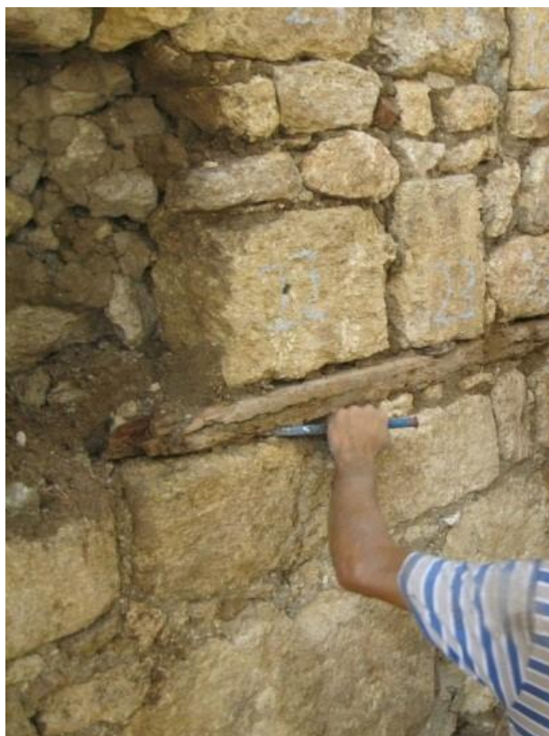
Figure A. 1. Removal of the Stones and Wooden Lintels (Source: SAYKA,2025)
