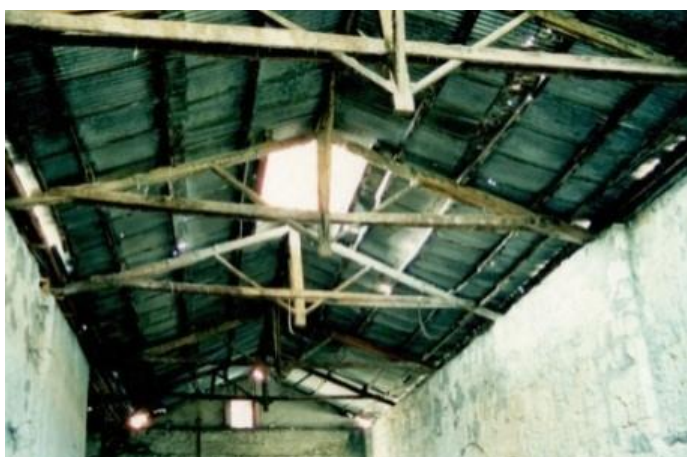
Figure 40. Original Roof Trusses of the Building B (Source, 2025)
