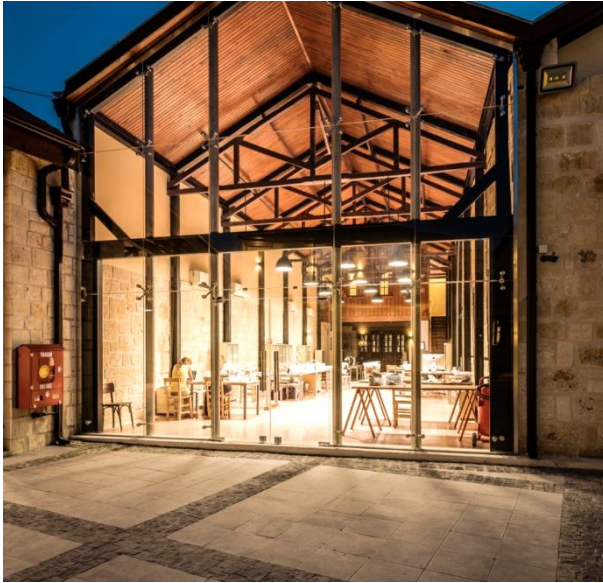
Figure 47. Spider glass cladding facade system of open work area in Building A, view from courtyard. (SAYKA,2025)
