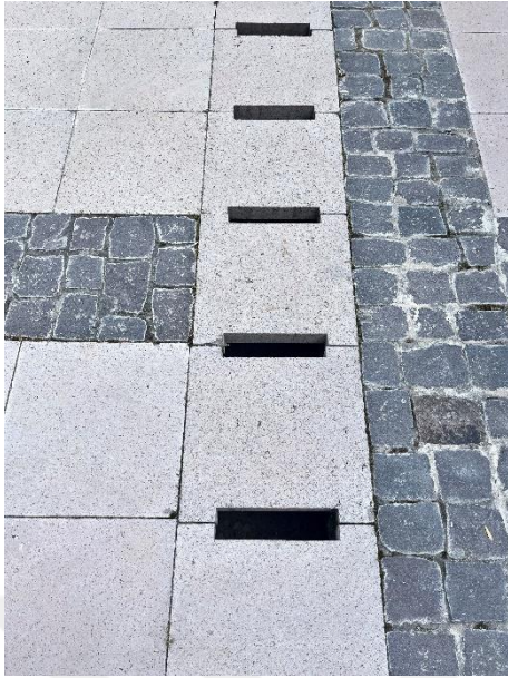
Figure 36. New Floorings of the courtyard
