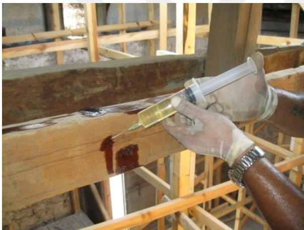
Figure A. 5. Reinforcing the wooden trusses with injection method (Source: SAYKA, 2025)
