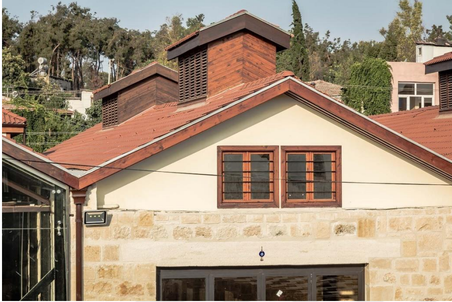
Figure 19. Roof Lanterns on the roof of Exhibition Hall in Building A (Source: Arkiv, 2025)
