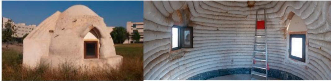
Figure 28. Earthbag building application, University of Lleida Campus, Spain (Rincón et al., 2020).
