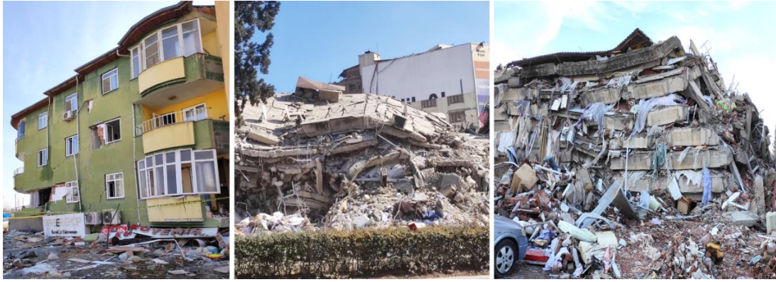
Figure 5.28 : Field reconnaissance images for soft-weak storey and pancake collapse mechanism
