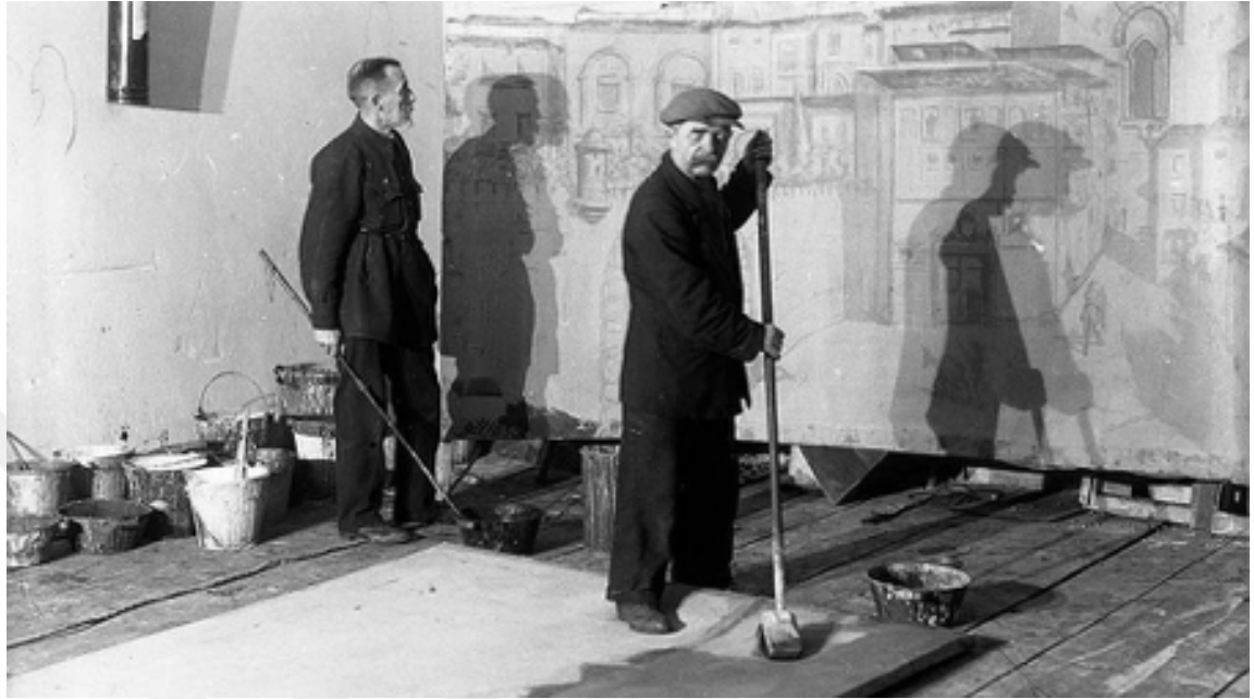
Figure 2.113. Installation of partitions in a Moscow apartment Russian State Film and Photo Archive (RGAKFD / Rosinform)
