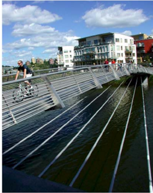
Figure 1.3 : The Apate Bridge,
