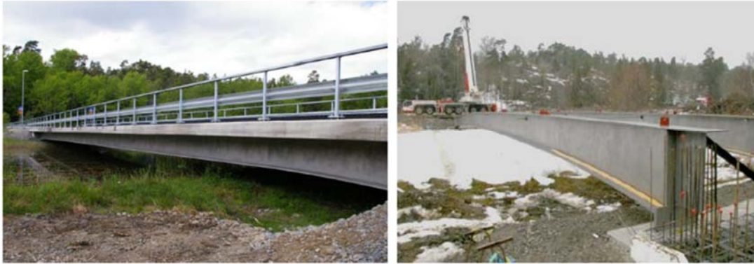
Figure 1.5 : One of stainless beams of the load bearing structure.
