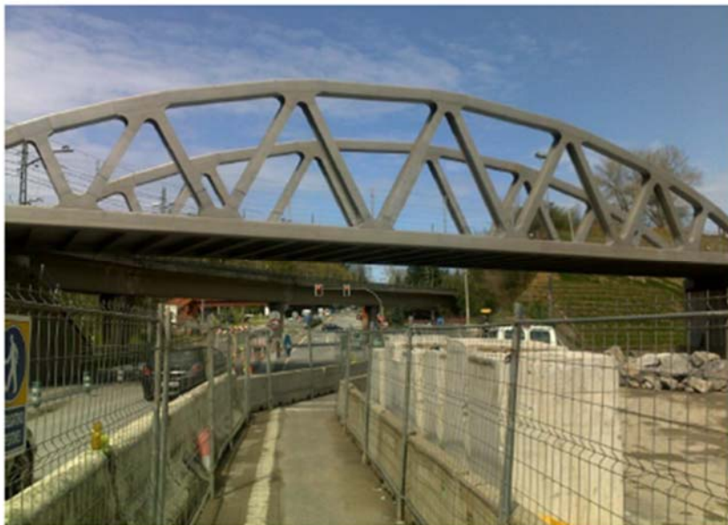
Figure 1.6 : The entire truss structure
