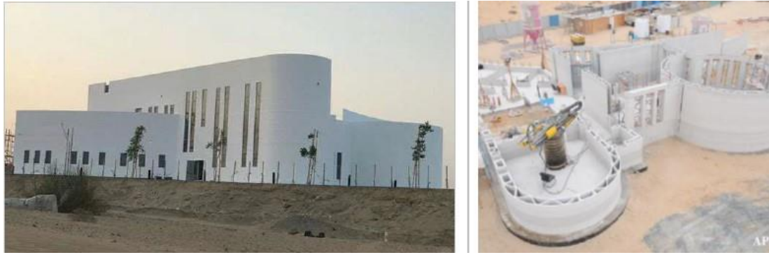
Figure 2.6 Dubai Municipality Office printed by Apis Cor.
