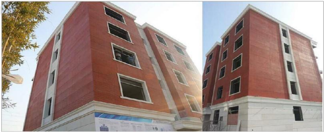
Figure 2.5 WinSun company printed 5-storeys building.
