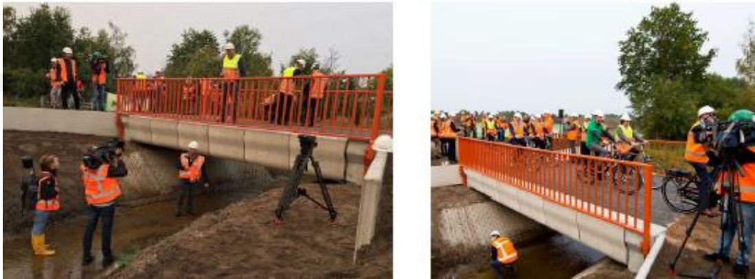
Figure 2.8 3D printed bicycle bridge in Netherlands [12].
