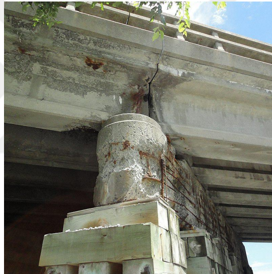
Figure 1.2. Exemplification of Expansion Joint Leakage Issue.
