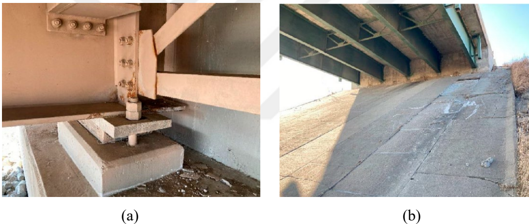
Figure 1.1. Connection between bridge superstructure and abutment of: (a) a traditional bridge and (b) an IAB.
