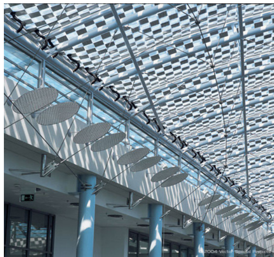
Figure 4.6: Roof structure of atrium space; ETFE Foil cushion
