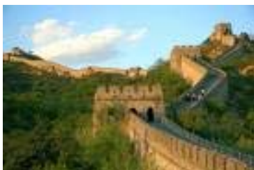
The Great Wall of China ...
