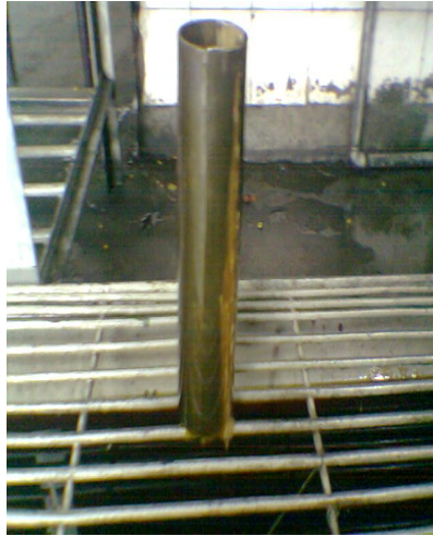
Figure 3.1. Piece of oily and rusty pipe specimen.
