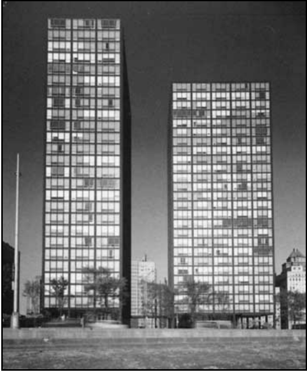
Şekil 2.1.3.2.: Lake Shore Drive Apartments
