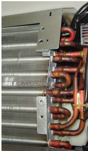
Figure C.1 : Indoor unit tube circuits, a) left view, b) right view
