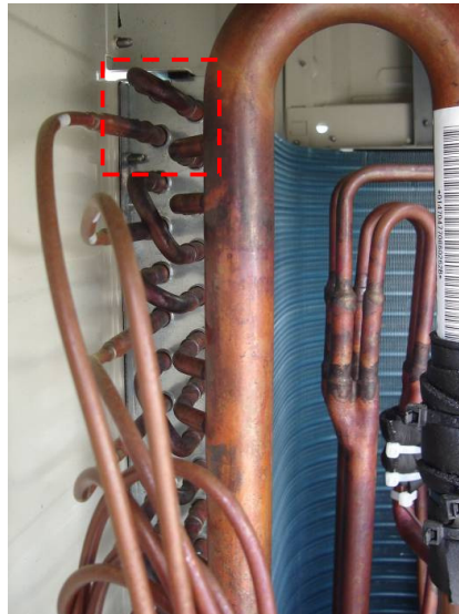
Figure C.5 : Outdoor unit tube circuits
