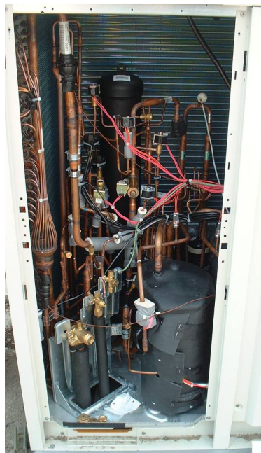
Figure 4.4 : Inside of the outdoor unit
