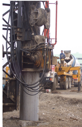
(d) Casing is withdrawn
