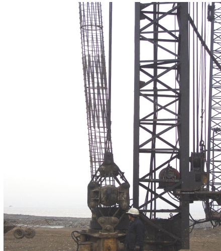
(c) Installation of the reinforcing cage
