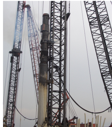
(b) Installation of steel casing
