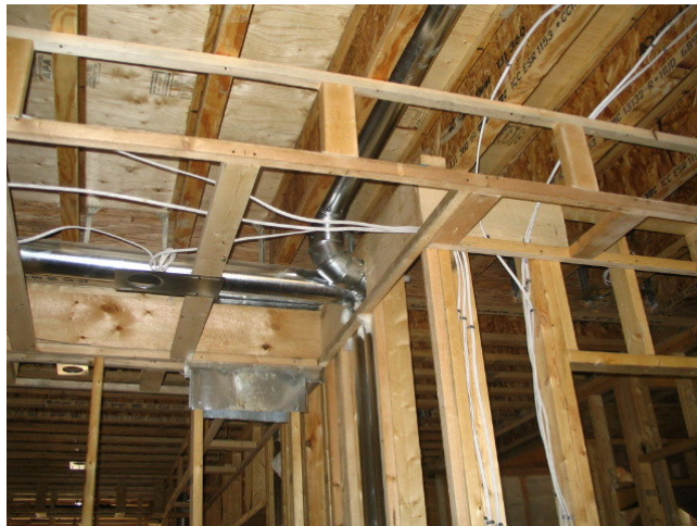
Figure 4-11: Framing Details for Heating and Electrical Cables.
