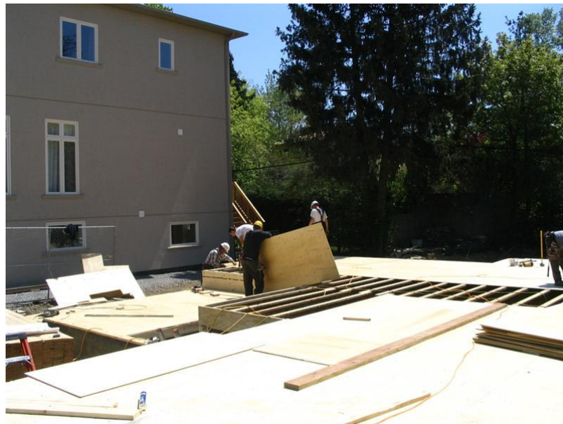
Figure 4-5: Installation of Floor Sheathing.
