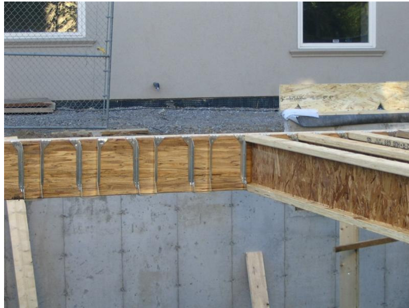
Figure 4-4: Joist Hangers.
