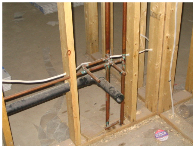
Figure 4-9: Framing Details for Plumbing.
