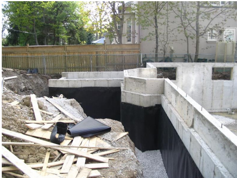
Figure 4-1: Foundation Walls right before backfilling.
