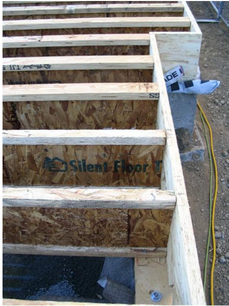
Figure 4-2: Sill Plate and Floor Joist detail.
