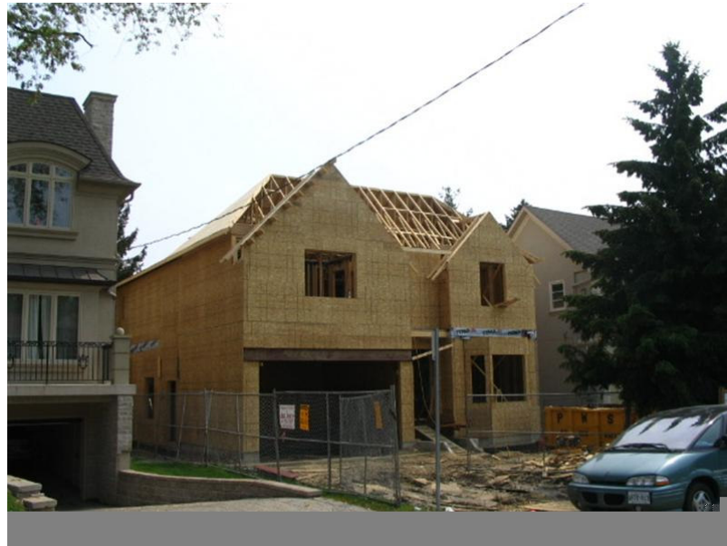
Figure 4-8: Roof Trusses.
