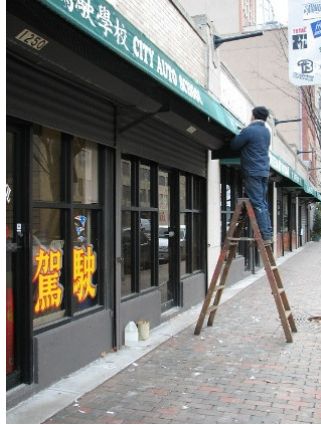
Figure 40. Maintenance of the street
