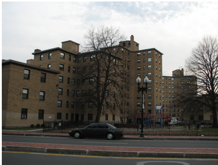
Figure 17. Cathedral Housing Project located on Washington Street: Housing Developments built after urban renewal. (December 28, 2005)
