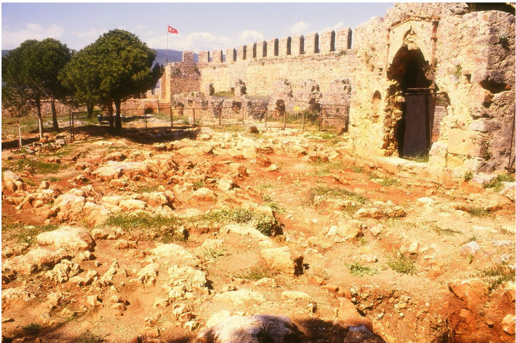
Figure 10: Vaulted (Tonozlu) Galleria
